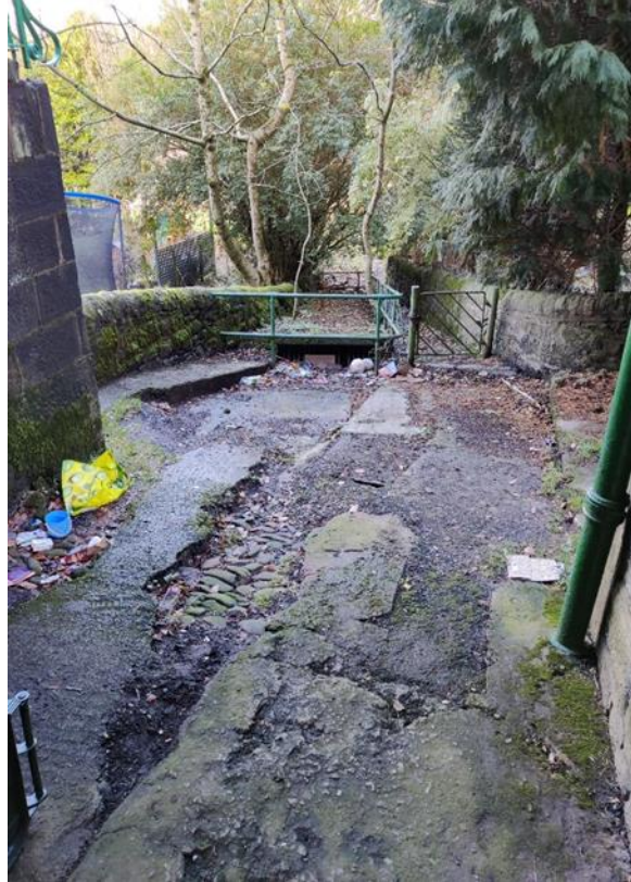
Figure 5: Overland flow capture inlet near Hey Top houses
